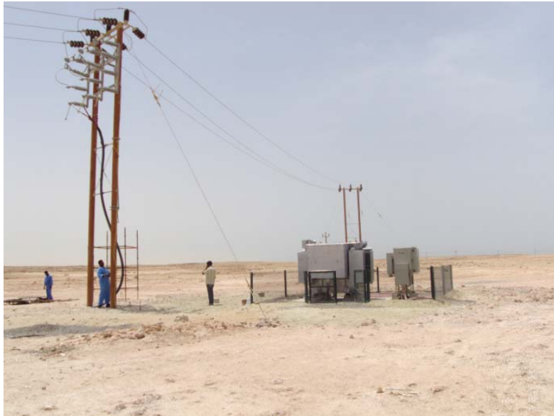
11kV Overhead line installation, Under ground cable pulling, transformer installation
